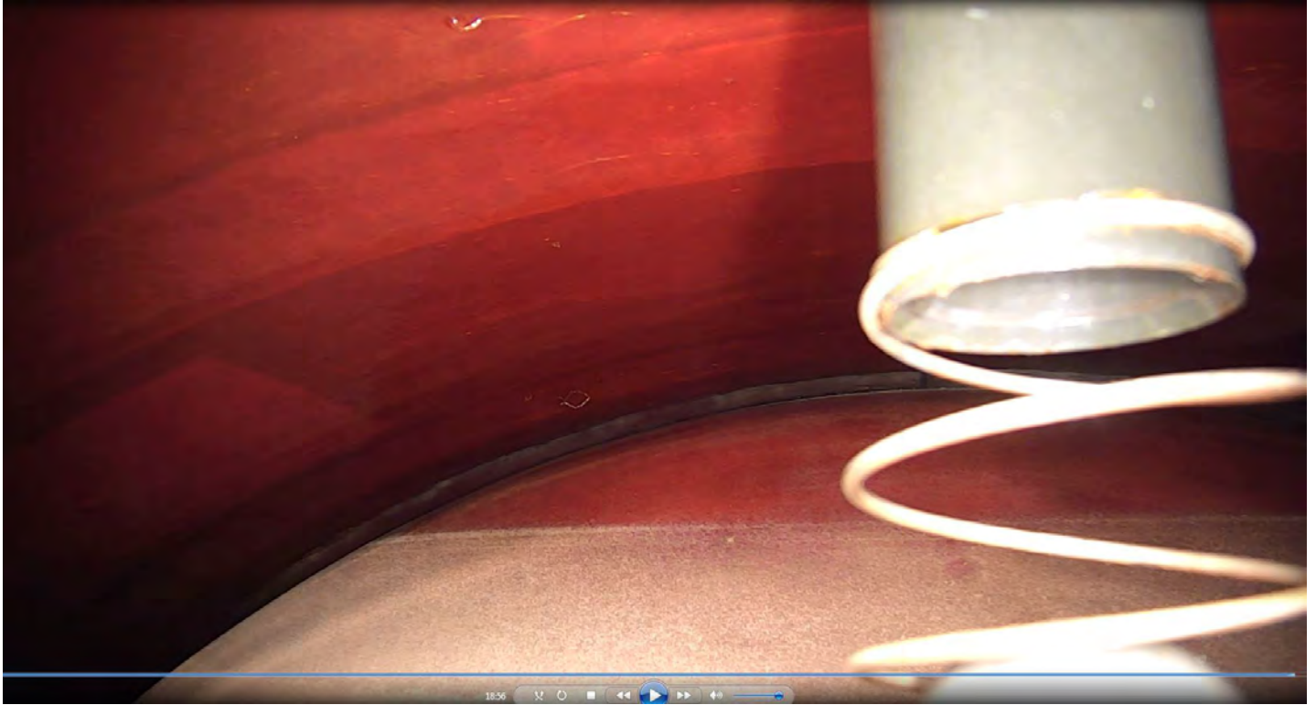
Figure 3-11: Top of end dome (18:56)
