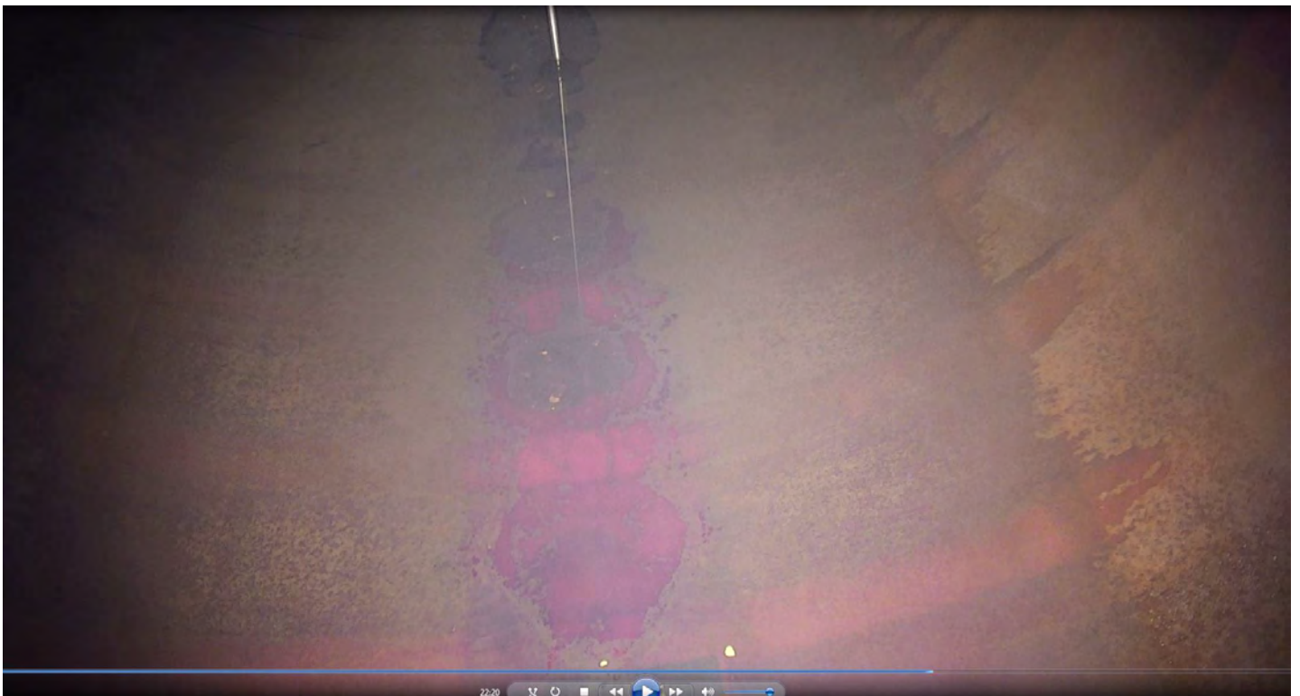
Figure 1-6: Sediment/residue on tank bottom (22:20)
