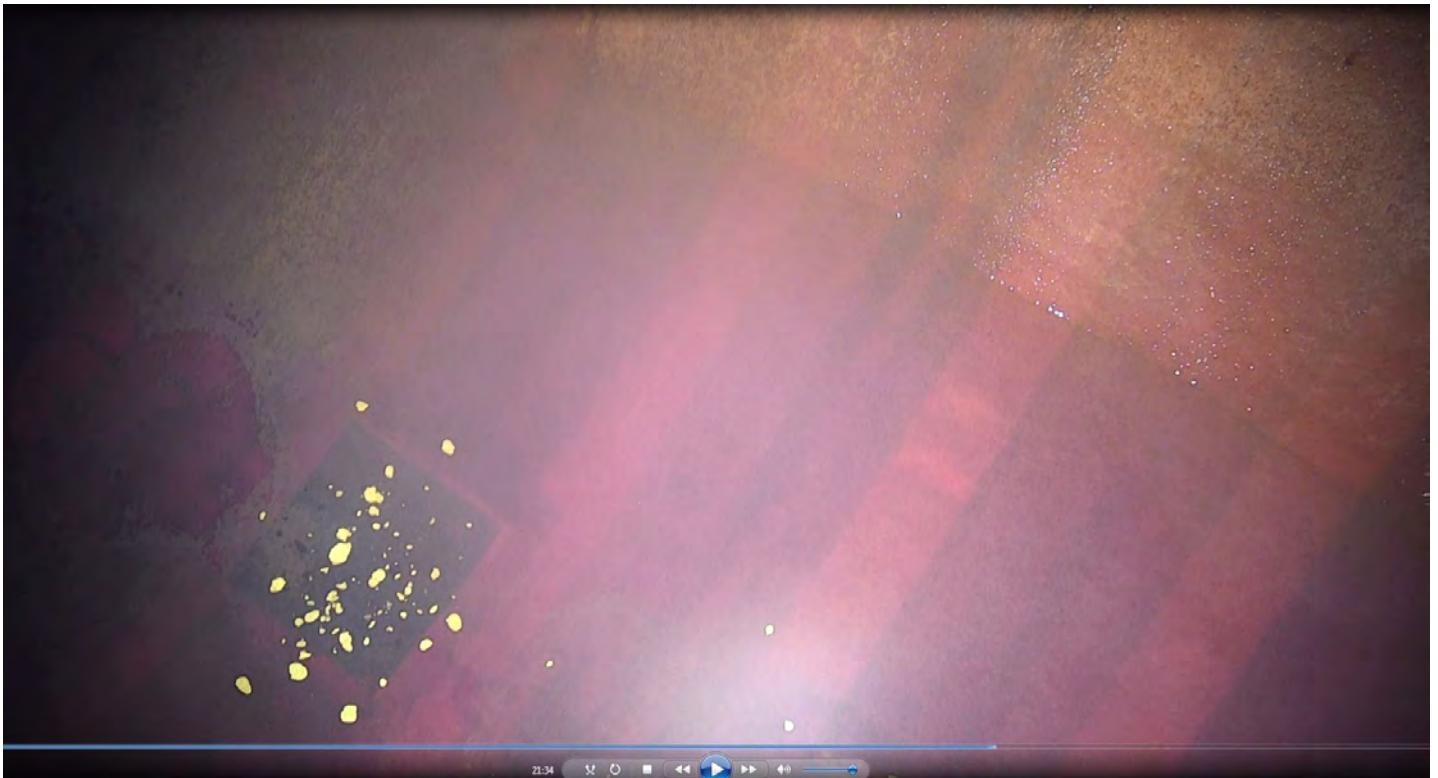
Figure 1-7: Possible gravel on tank bottom (21:34)
