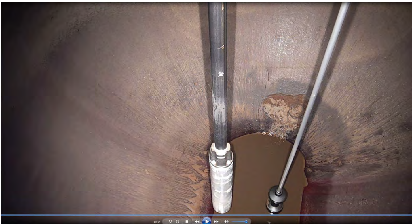
Figure 3-2: Sediment/residue on tank bottom (19:32)
